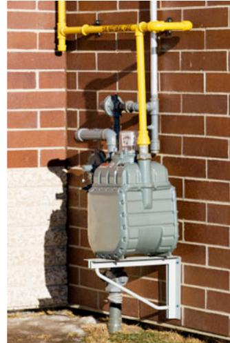
Gas is a versatile fuel that can be stored in underground reservoirs, in pipes and in tanks. It can be converted easily to a pressurized form known as liquid propane gas (LPG) and made available to those living far from pipelines. Underground pipes deliver natural gas to building foundations for consumption. From there, gas is sent through a metering device and delivered through tap-offs to any gas appliance. The meter is read periodically in order to bill consumers.
